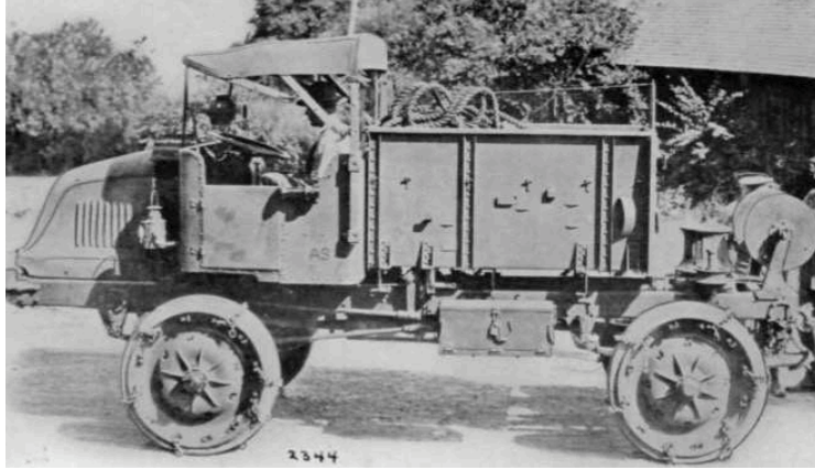
The artillery tractor variant of the Militor showing the power-driven winch on the back. (Field Artillery Journal Photo)
